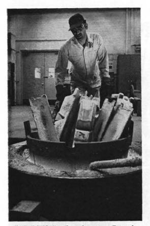
"CHARGING" the furnace, Damacio Sandoval watches aluminum ingots slowly sink into a white-hot gleaming mass. Giant crucible holds 900 lbs. of casting metal.
